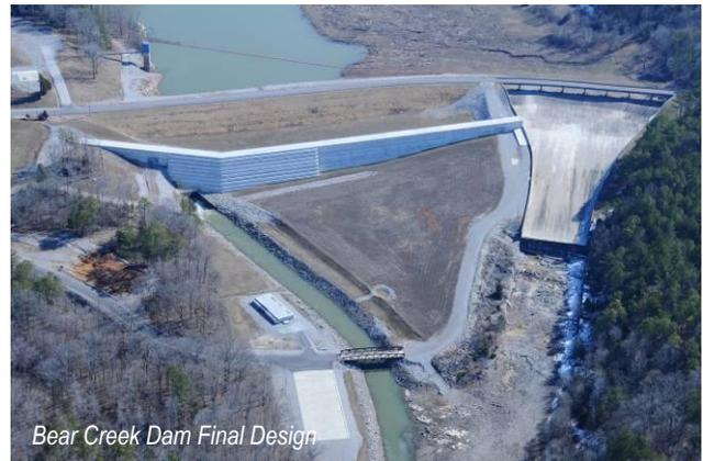
**DESIGN ENGINEERING:** RIZZO personnel performed a comprehensive subsurface investigation and subsequently developed all design details, drawings, and specifications for the composite seepage barrier and RCC berm from initial through final design.
