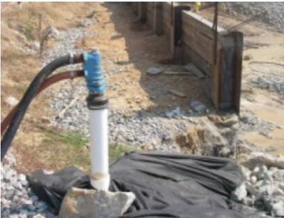
RIZZO designed the excavation and associated deep well dewatering system for the Smithland Hydroelectric Power Plant Facility currently under construction on the Ohio River in Kentucky. To support the design, RIZZO conducted pumping
