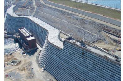
Work on the Saluda Dam Remediation Project earned RIZZO ASCE's prestigious Outstanding Civil Engineering Opal Award in 2006. Additionally, during production of the middle third of the dam, the RIZZO team set the new North American Industry RCC Placement Record, placing 18,590 cubic yards of RCC in a 24-hour period.
