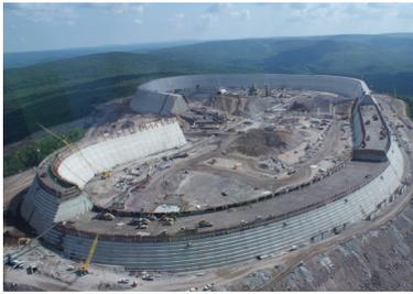
RIZZO evaluated several alternatives for a re-build and selected a symmetrical section, Roller Compacted Concrete (RCC) Dam. The symmetrical slopes reduced the demand on the rock foundation and allowed for the use of aggregate recycled
